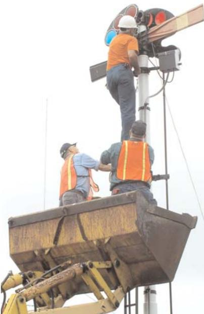
grinding and sand blasting to restore it to usable condition. In addition the two rigid sheet metal frames (called spectacles) which support the colored lenses, were worn beyond repair and had to be duplicated. Both the repair and the replacement work were performed by Gary Herrmann, Gerry's son. This highly technical work was the only work contracted out during this restoration.
