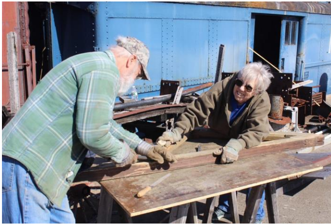
DON KONEN AND PATTY OSMER SCAPING SUPPORTS
