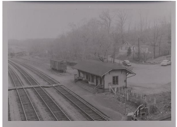
Cruers, NY Station April 1956
